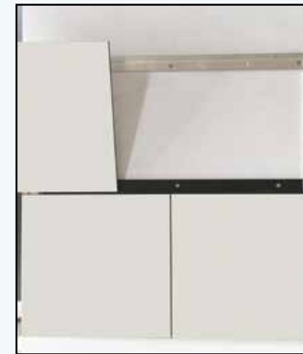
Step-1:- Bottom half of the Shaurya is already installed, installation of upper half is about to start.
