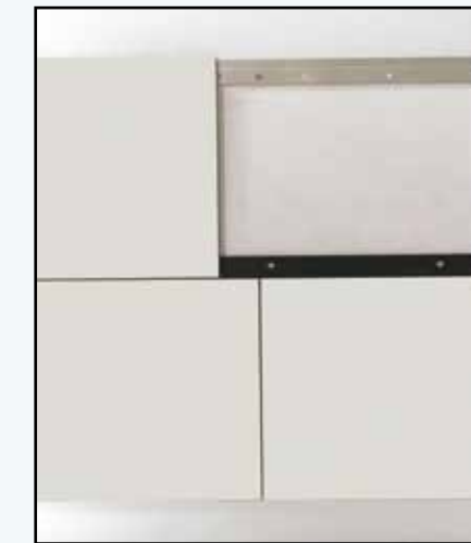
Step-2:- First Merino HPL compact panel is getting mounted on the profile.
